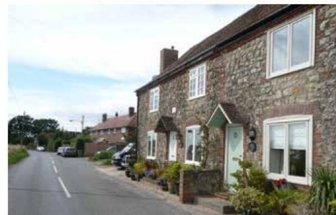
Local Greensand and Kentish Ragstone in the older buildings of Lympne, Aldington and Westenhanger
